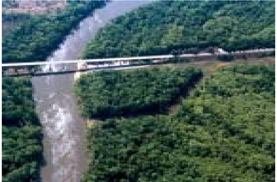
US 601 bridge over the Congaree River.
