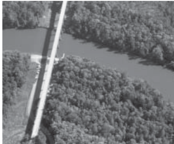
US 601 bridge over Congaree River.
