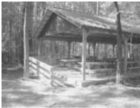
New picnic shelter
